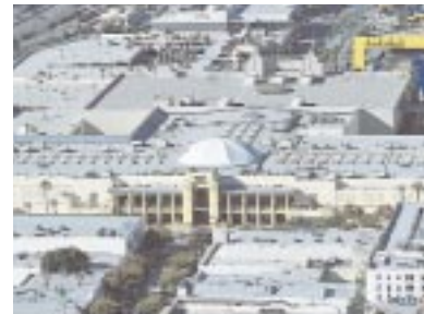
MEDIA CITY REGIONAL SHOPPING CENTER Burbank, CA Architect: Bastien and Associates/ Stoutenborough, Inc. and Leason Pomeroy Associates
