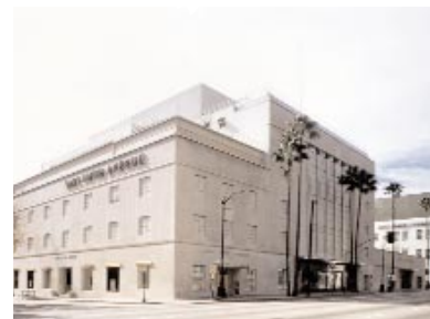
SAKS FIFTH AVENUE EAST AND WEST Beverly Hills, CA Architect: Bridges Lavin and HTL/Space Design International
