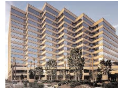
SONY (COLUMBIA) PICTURES Burbank, CA Architect: Gensler and Associates
